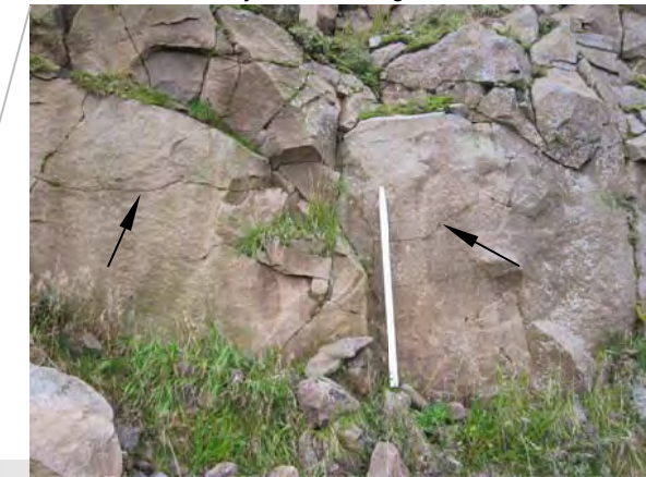
Typical massive basalt observed on quarry face. Note random fractures indicated by arrows throughout the rock mass
