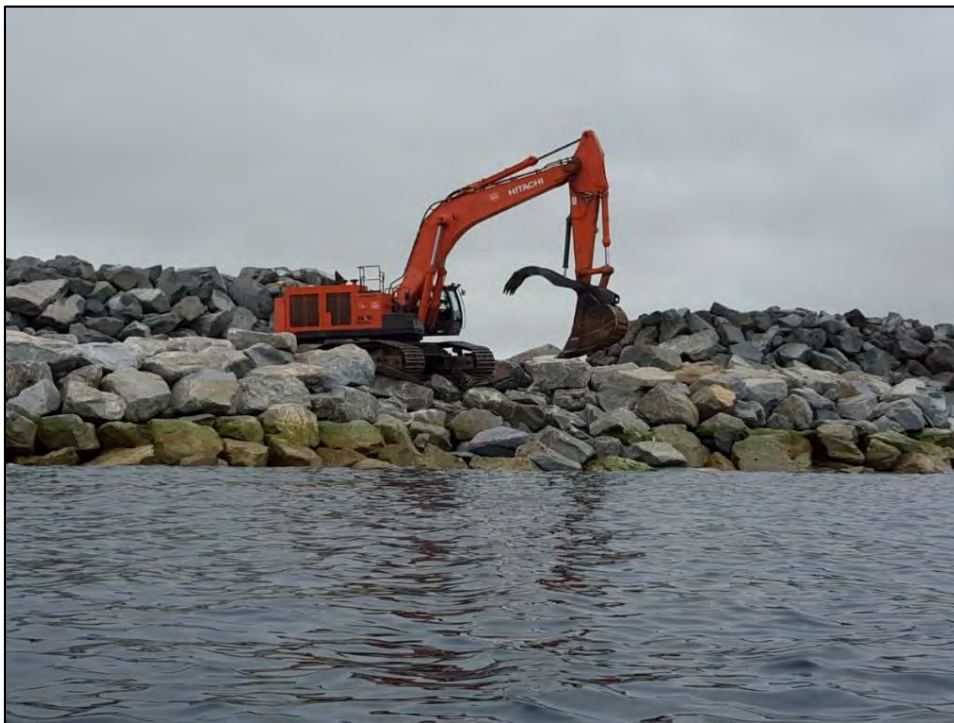
Figure C-10. Locking Armor Stone into the Breakwater
