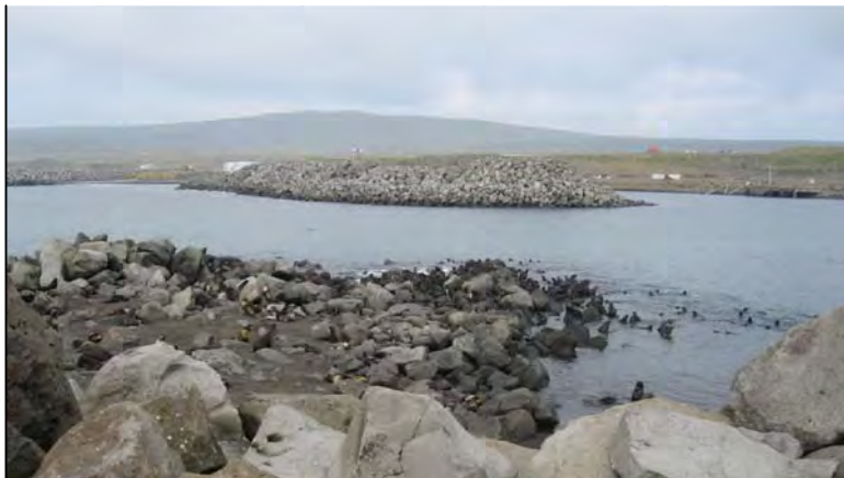
View of Inner Breawater from South Breakwater, St. George Harbor
