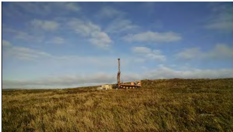
Drilling Boring B-8 Near Maynard Hill, Airport Rock Quarry
