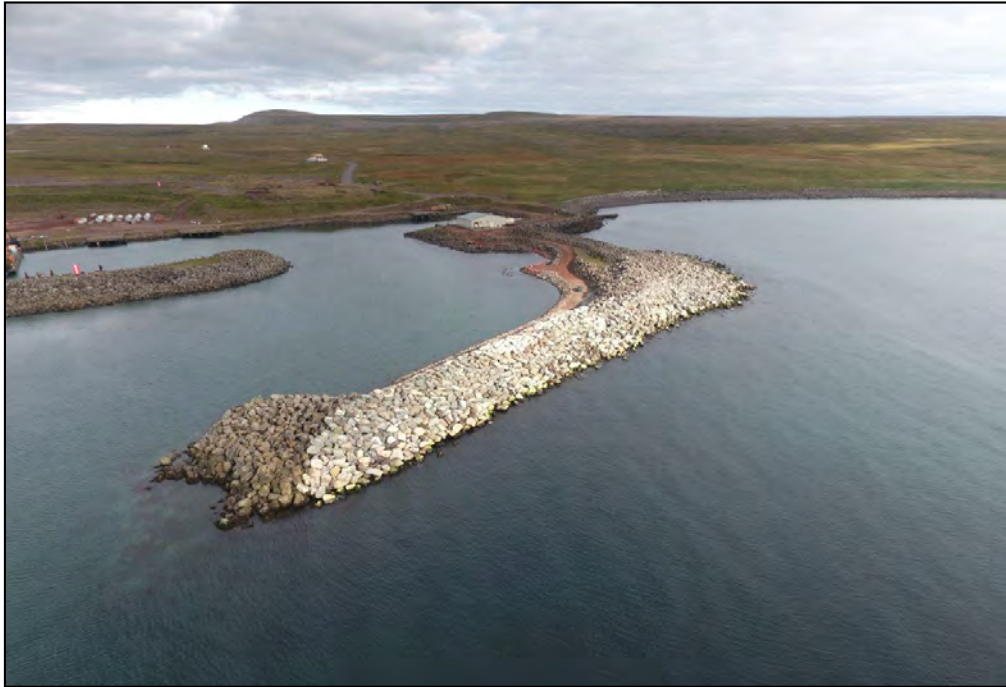
Figure C-6. Breakwater after Repairs, 2017
