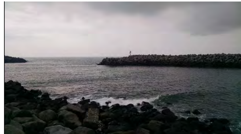
View of North Breawater from Inner Breakwater, St. George Harbor
