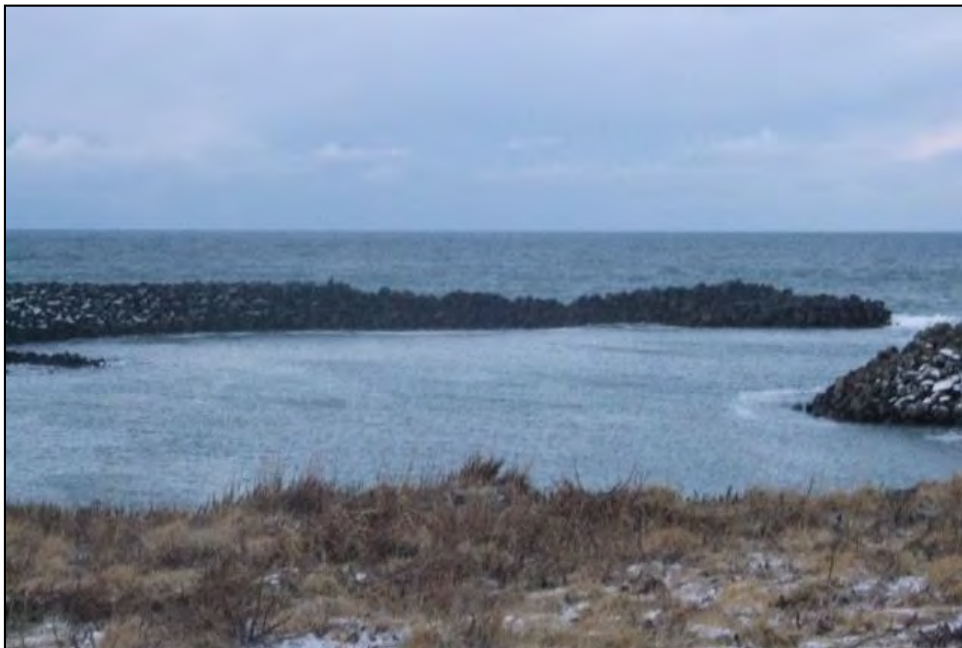
Figure C-5. Breakwater after December 2015 Storms
