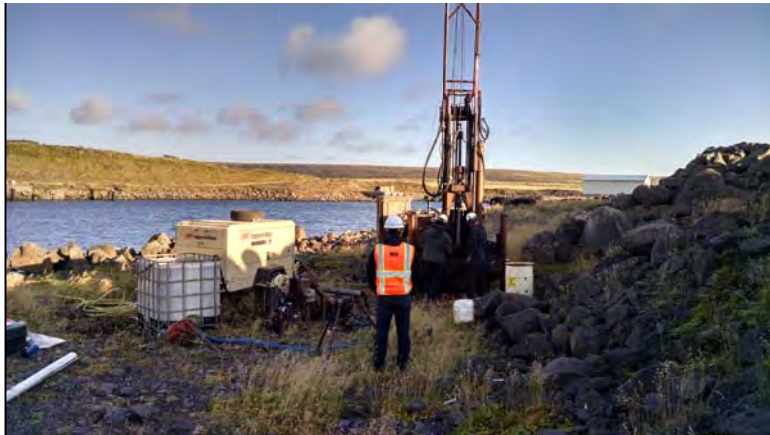
Drilling Boring B-3 on Inner Breakwater, St. George Harbor
